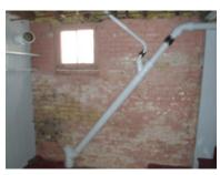
PVC-rigid plastic pipe (generally white in color). There is also some cast iron piping installed.
